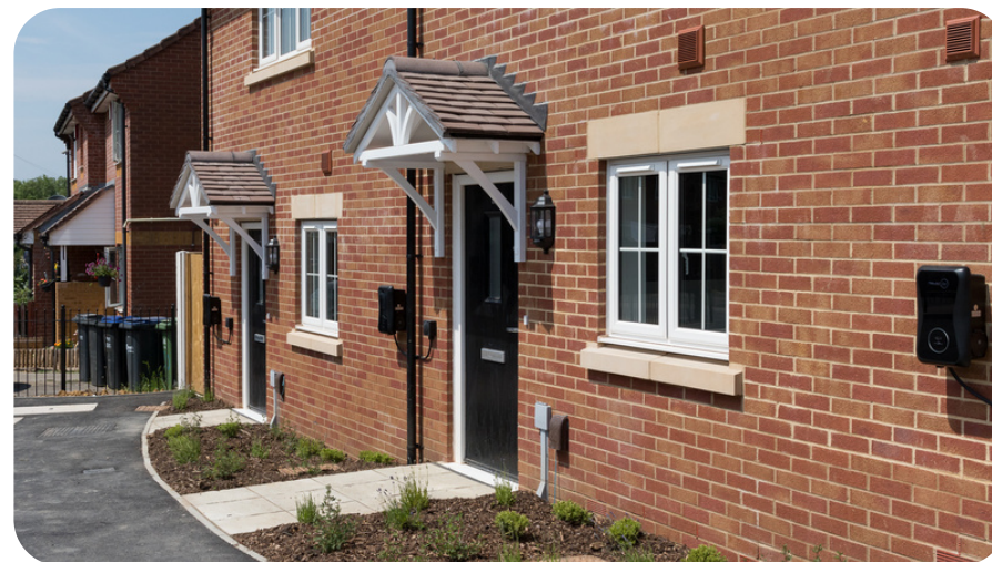
New EPC 'A' rated homes completed on the site of the derelict John Bull pub in Trowbridge.
